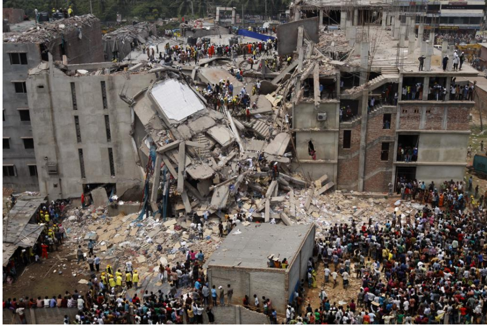
Figure 2: Rana Plaza building collapse
